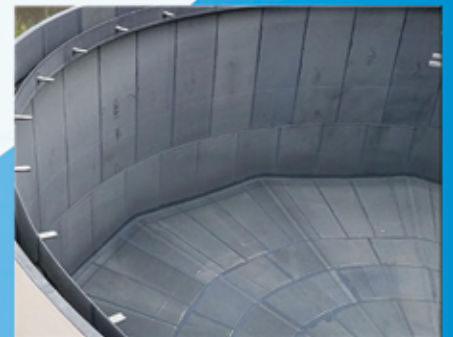
RUBBER LINING INSIDE STORAGE TANK
