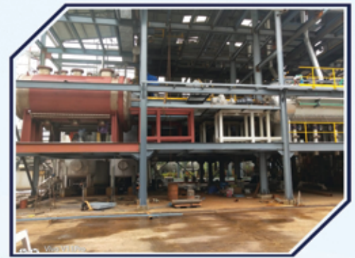
Project at Haldia
