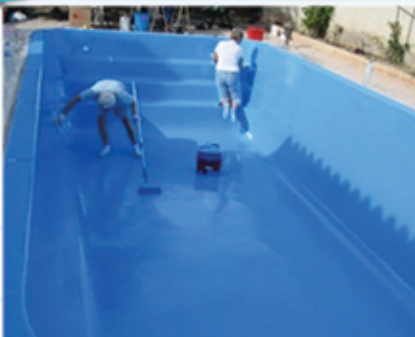
FRP LINING IS IN PROGRESS
