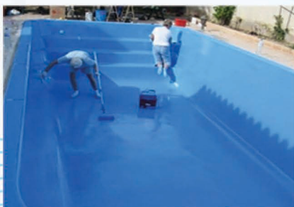
FRP LINING IS IN PROGRESS
