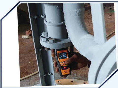
Dew Point Testing
